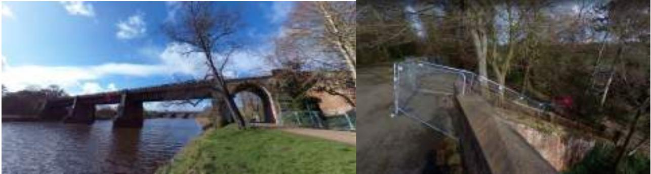
Figure 2-16: Avenham Viaduct bridge, left, with damaged staircase and footpath posing risk to the structure, right
